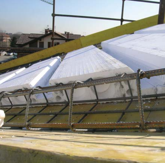
Roofing of a new building
