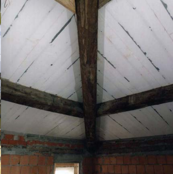
Roofing of a historic building
