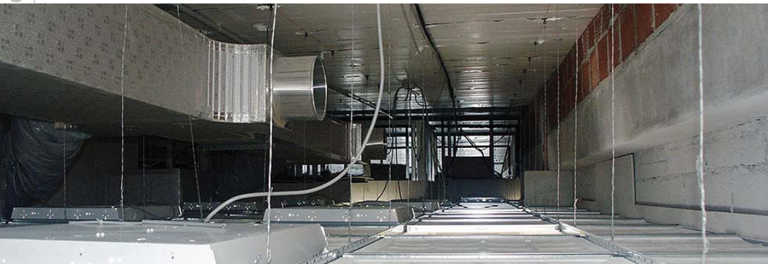
Lowered and dropped false ceiling
