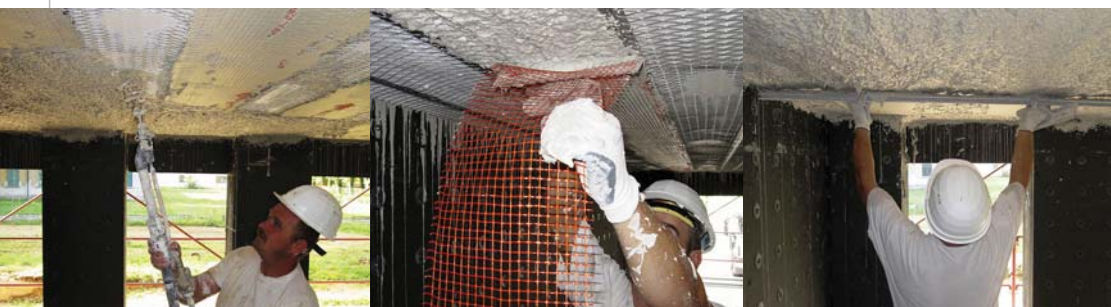
Laying of the machine
