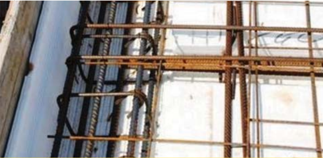
Laying of the balcony
